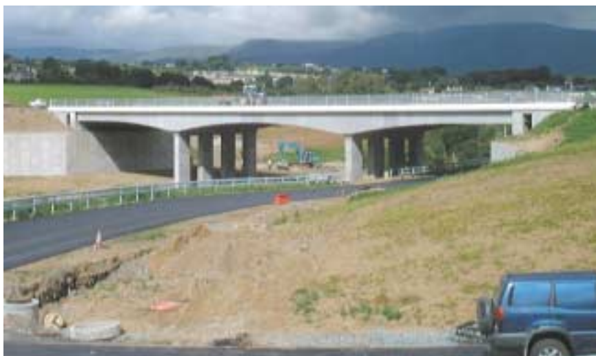
The Kilmacthomas bypass, Waterford.
