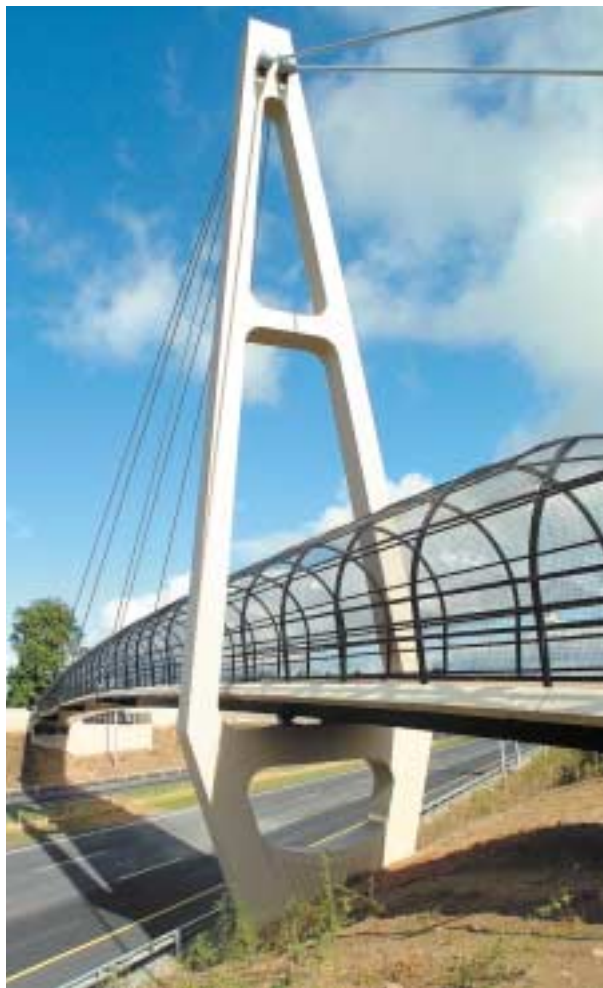
Footbridge over the M50
