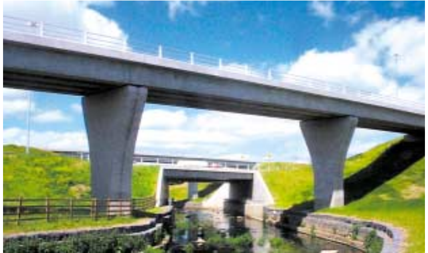
The Dunleer-Dundalk Motorway
